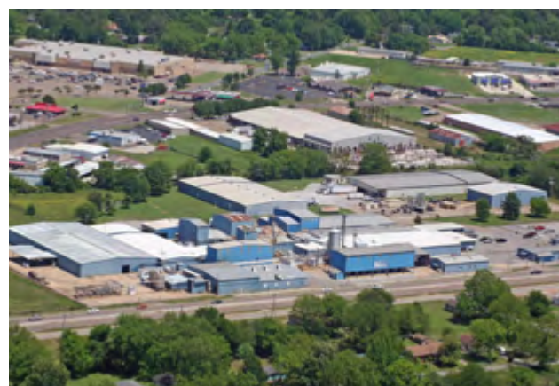
Production Facility of Helena Group (AR, U.S.)
