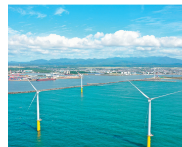
Offshore Wind Farm at Akita Port in Akita Prefecture (courtesy of Akita Offshore Wind Corporation)
