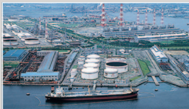
2 Petroleum product receiving and shipping terminal (Marubeni Ennex Corporation) (Japan)
