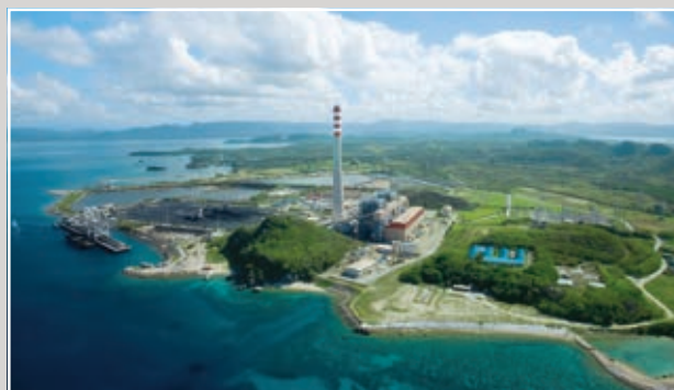
2 Pagbilao power plant (Philippines)
