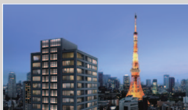
2 GRAND-SUITE Azabudai Hilltop Tower condominium complex in Tokyo (Japan)
