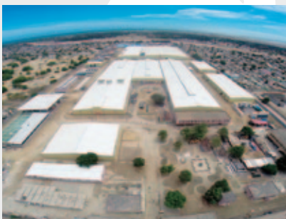
Textile factory rehabilitation project (Angola)
