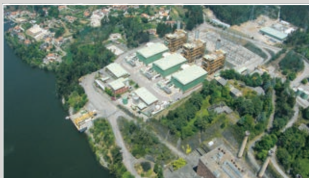
1 Turbogas combined cycle thermal power plant (Portugal)
