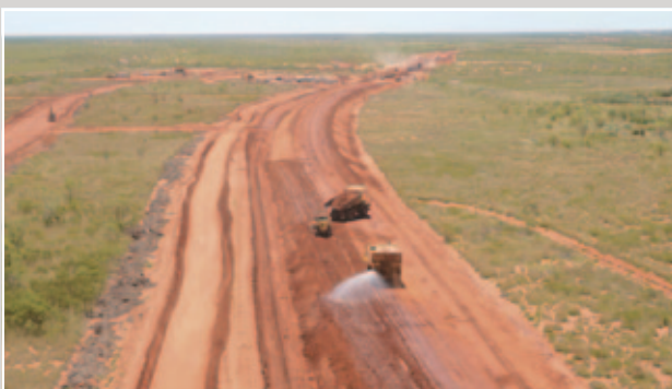
1 Railroad under construction at the Roy Hill Iron Ore Mine (Australia)
