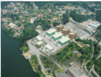
Turbogas combined cycle thermal power plant (Portugal)
