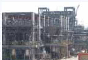
Synthetic rubber manufacturing facility (India)
