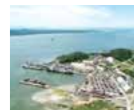
Export terminal of Terlogs Terminal Maritimo Ltda. (Brazil)
