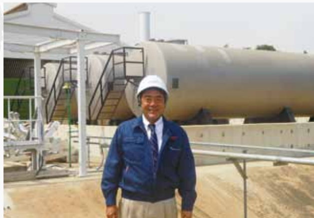
Mr. Nagashima at a plant under construction
