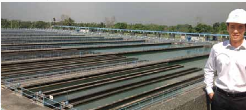
Mr. Ogawa at the Maynilad water purification facility
