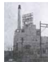
Unit No. 1 at Manila Electric Company (Philippines)
