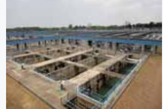
Maynilad Water Services, Inc. La Mesa Water Treatment Plant (Philippines)
